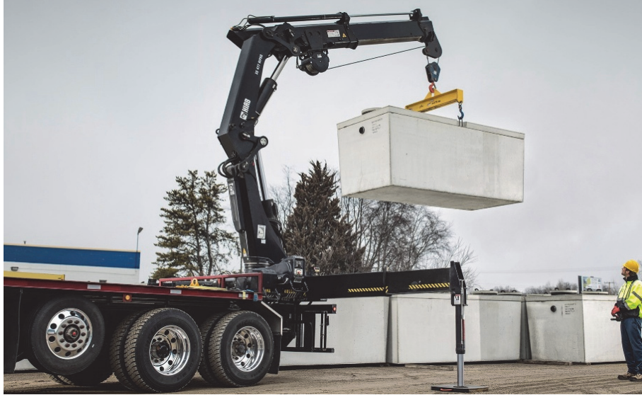
Figure 19 – Hiab truck places 2400mm pipe into the trench.
