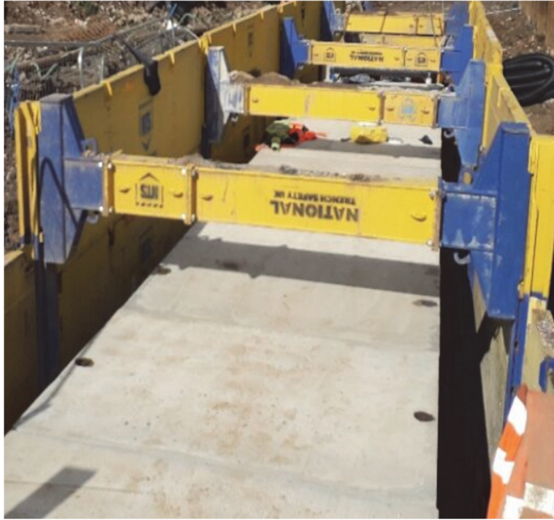
Figure 12 – Trench Box – Slide Rail System
