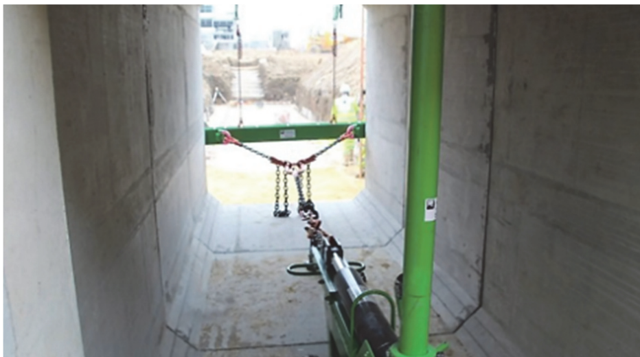
Figure 20 – Culvert Puller
