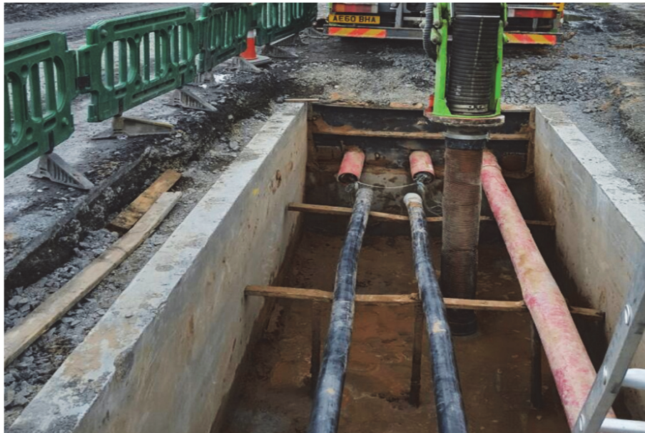
Figure 1 – Vacuum Excavation
