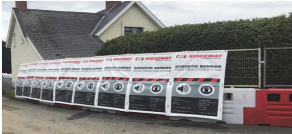
Figure 7 – Water filled barriers with acoustic blanket
