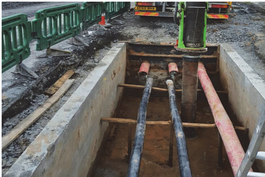
Figure 1 – Vacuum Excavation
