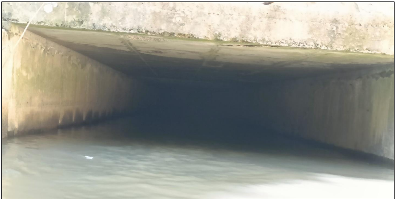
Figure 5-6: Culvert running under the N11 that heads to the Bray Road site and Cherrywood Park
