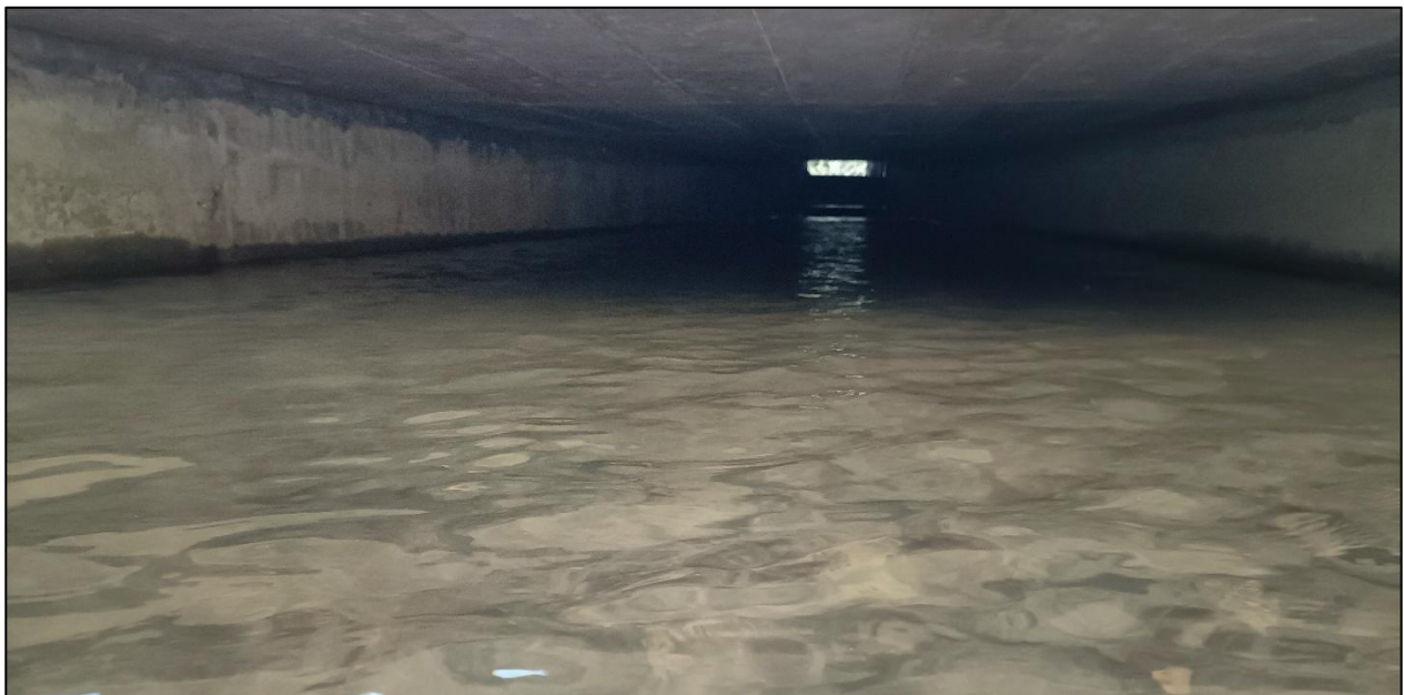
Figure 5-7: Culvert running under the N11, far end is stream that goes to Cherrywood Road
